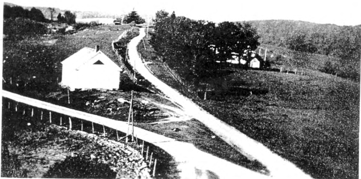
The Town Hall in an undated photograph, showing the roads dividing to East Craftsbury and to what is now T/H 8, with the Albert Cook property on the right.
