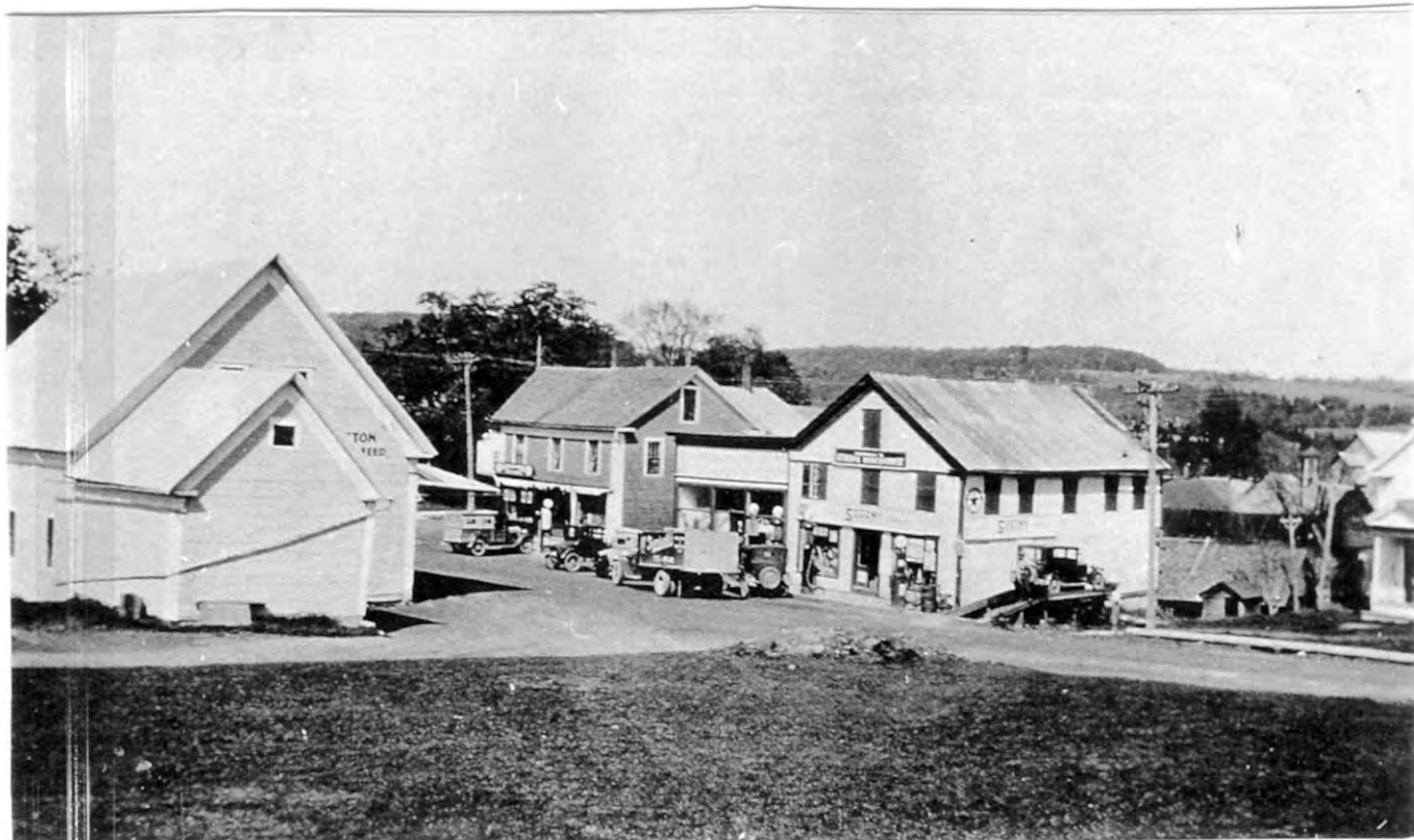
Note the gas pump and ramp for changing oil in front of the building on the right.
