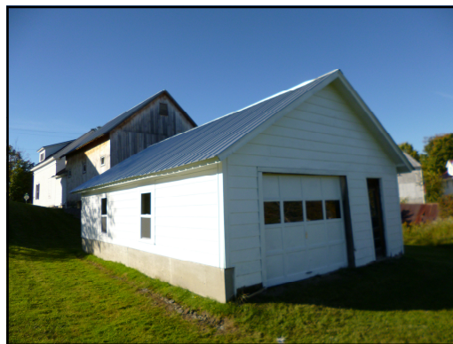
GHS shed with new roof and paint job
