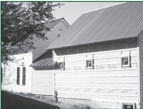
East side of building, showing how the barn complements the original building 5-15-10.
