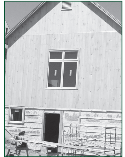
The rear of the GHS barn & entry to archives and work space on lower level 5-22-10.
